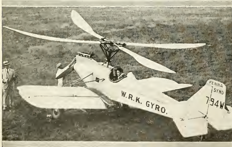
The Wilford gyroplane with rigid rotor blades having a span of 25 feet
